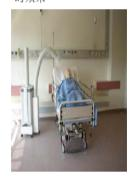
The Outflow duct should not be placed near the air supply
